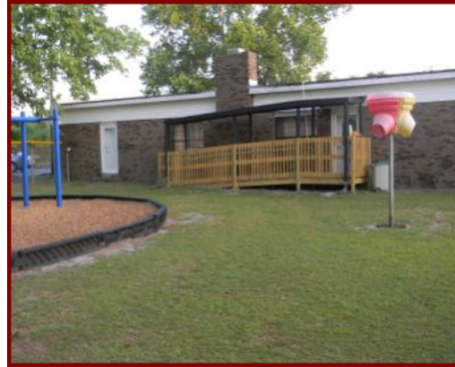
B.W. Lester Center had a new handicap ramp directly accessing the playground.
