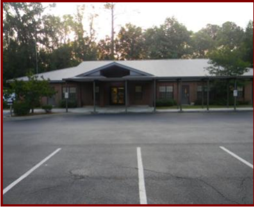
Hallmark Heights Center in Valdosta received a new metal roof.
