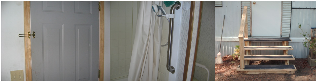
Door frame repair for safety
